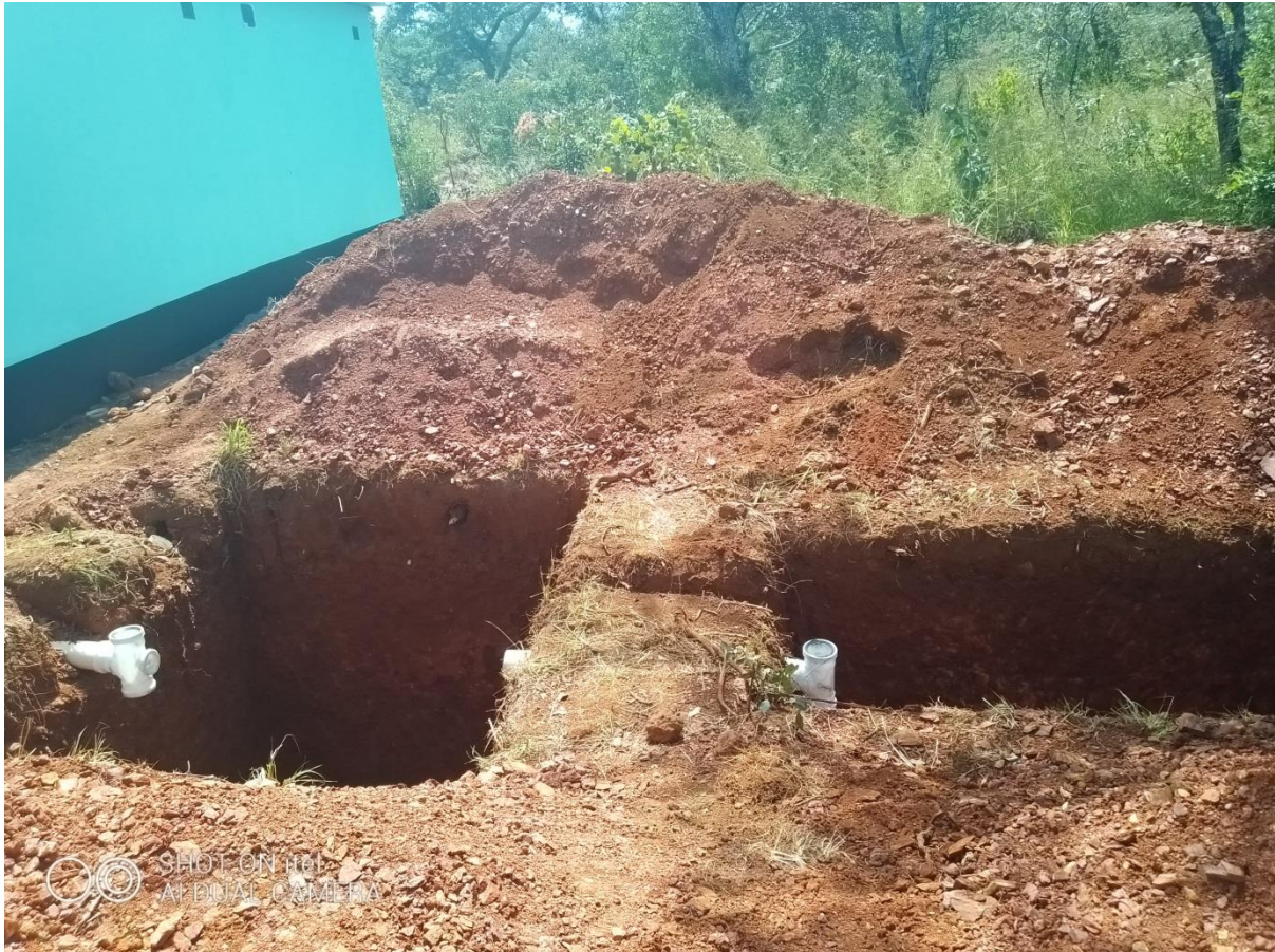
A small septic tank awaiting construction
