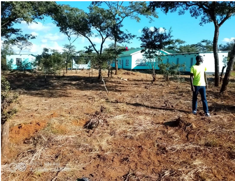
The final outlook. The kitchen, hostel, classrooms and cottage were painted successfully. Trees shall be maintained to enhance a serene environment.
