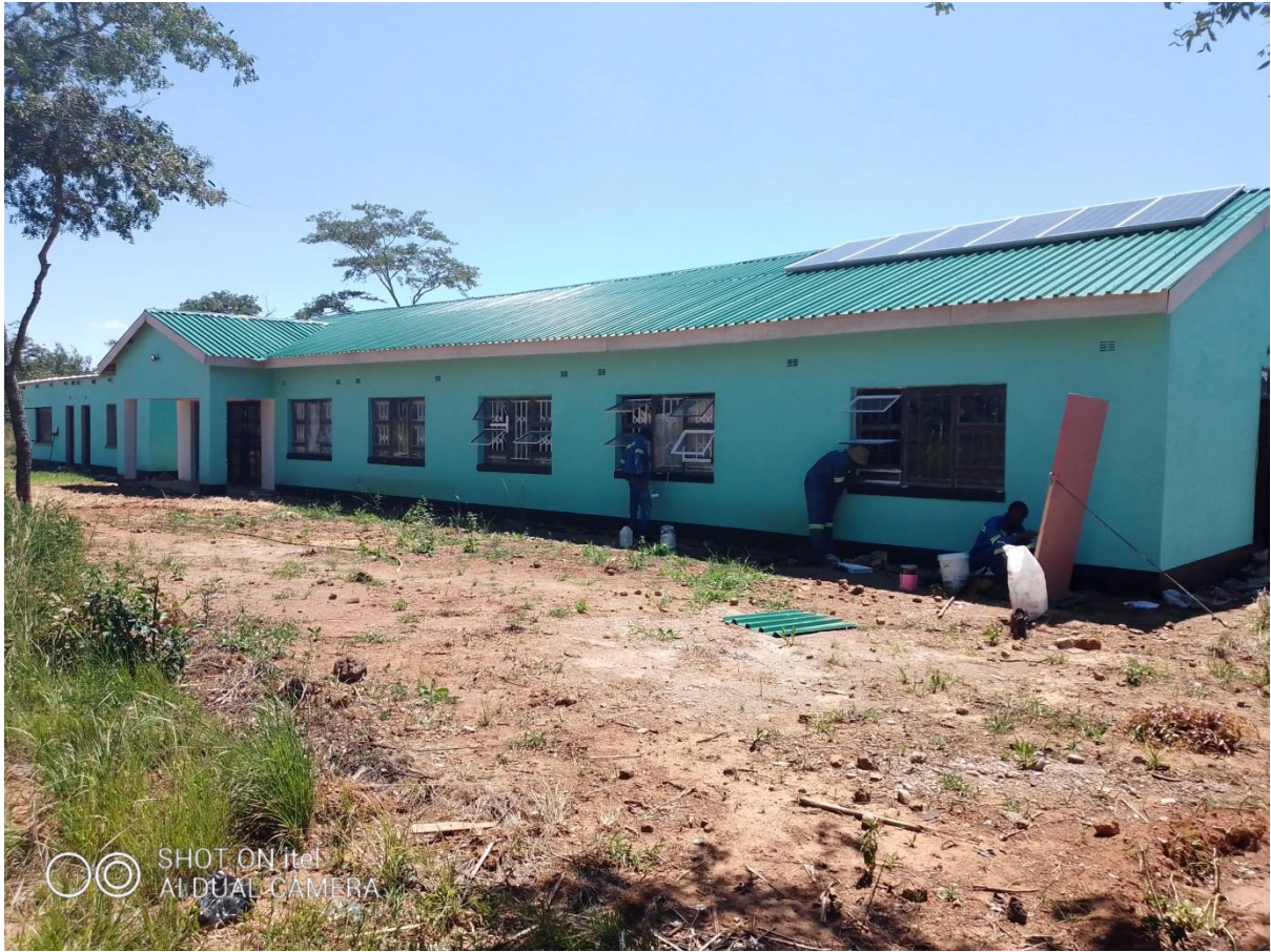
Final touch-ups on the walls (painting) being done on the hostel
